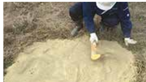
⑥ Make even or smooth with a small hand shovel after spraying.
