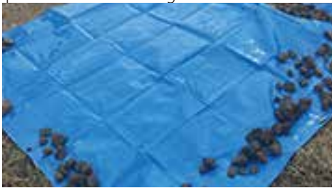
⑧ After work, cover the hole with a sheet to prevent unnecessary water like rain.
