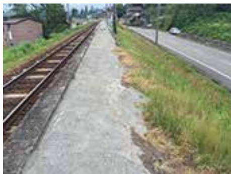
Used as a weed control for railway facilities
