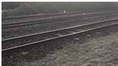
① Around the railroad, it takes some time to remove creeping weed in the vacant land.
